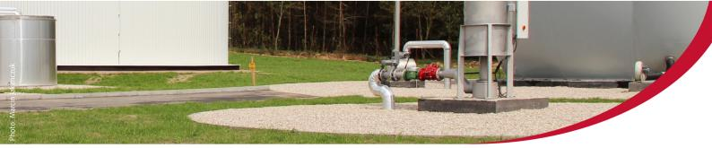
low-pressure tank. Then, through the pressure pump, biogas is transferred from the tank to the energy co-generation unit, where heat and electricity are produced. Heat is used to maintain process temperatures in digester chambers at adequate levels, while electricity is used for the wastewater treatment plant's own purposes. Each chamber is equipped with heat circulation system and doubleimpeller agitators, which ensure complete sludge mixing.
