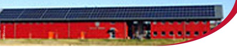
saves about 18 tonnes of CO2 and reduces power consumption from grid by 5%. Complete installed cost for is about 100,000 EUR. The plant contributed to improving the energy label of the building and gave experience with the installation and operation of photovoltaic plants.
